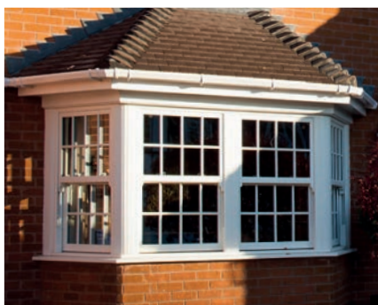
Bay window with vertical sliding sash windows
